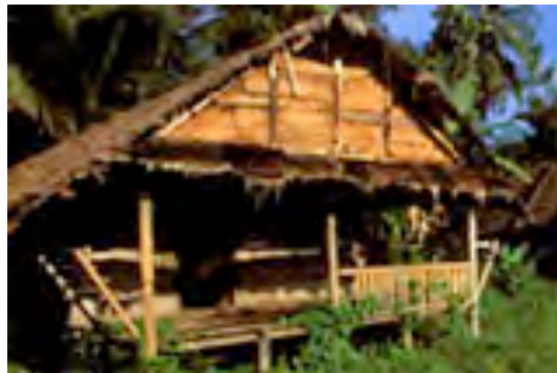
Building the umas or community houses will help the Metawai preserve their traditional culture. Credit: Native Planet
